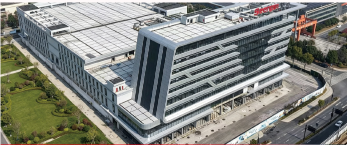
杭州新剑机电传动股份有限公司-总部、研发、制造基地大楼(杭州城西科创大走廊科技大道) Hangzhou Seenpin Electromechanical Transmission Co., Ltd.-Headquarters, R&D, and Manufacturing Base Building under Construction(Hangzhou West Science and Technology Innovation Corridor Science and Technology Avenue)
